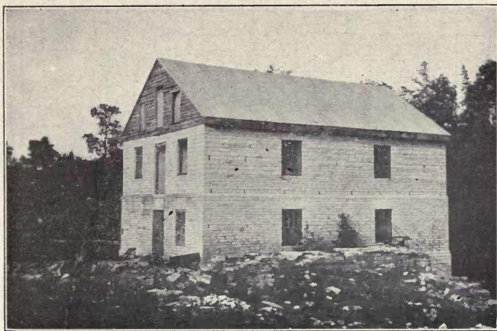
4. MORTON'S MILL, BOONE'S CREEK, FAYETTE COUNTY A structure with walls built of Tyrone limestone. Photograph by A. M. Miller
